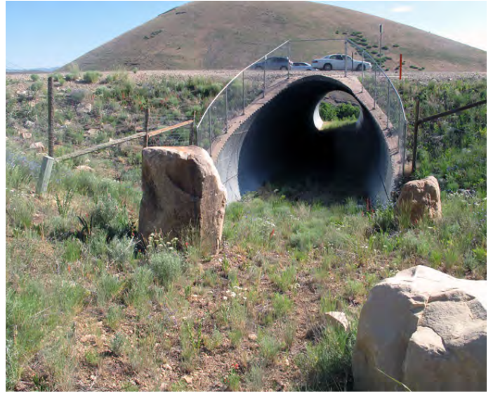
Deer Creek Culvert Underpass
