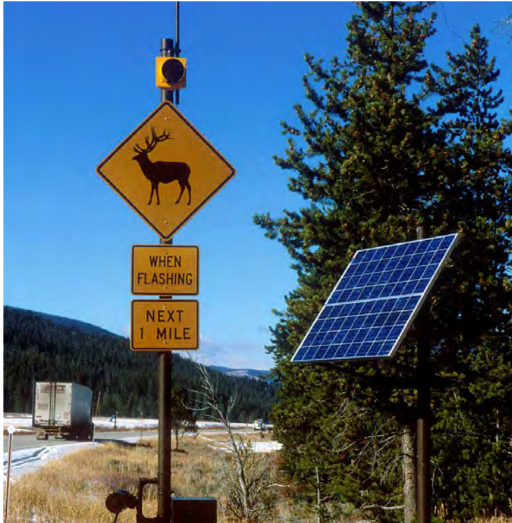
Animal Detection System on U.S. Highway 191
